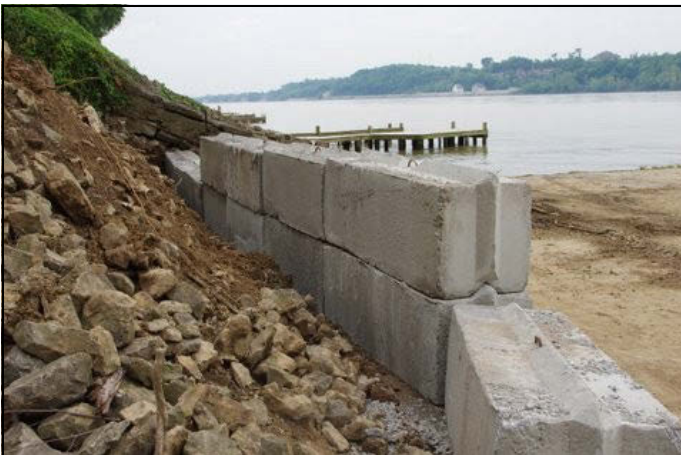
Looking downstream, LSC block project before completion.
