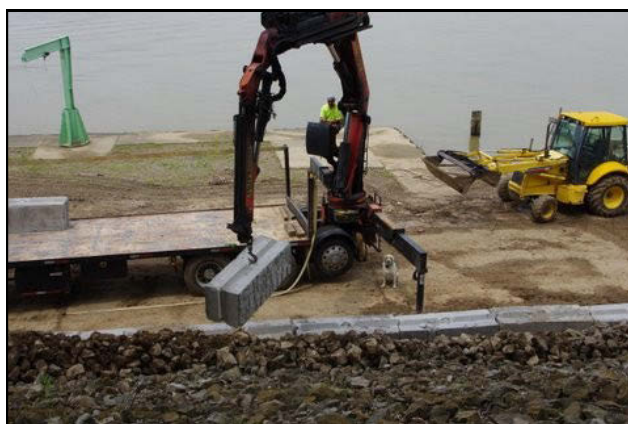
Putting improvements into place on LSC's lower level.
