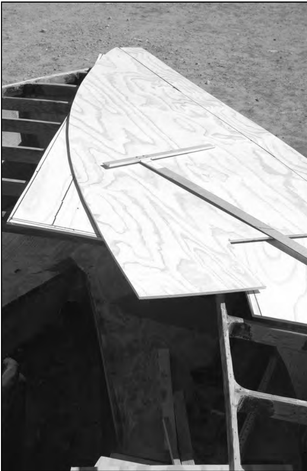
Cutting and fitting plywood deck, later in the project.
